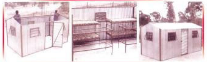
All panels are bolted together
